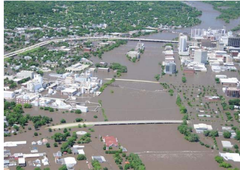
Figure 3. View of flooded Cedar Rapids in 2008, after a record flooding of the Cedar River. 12
